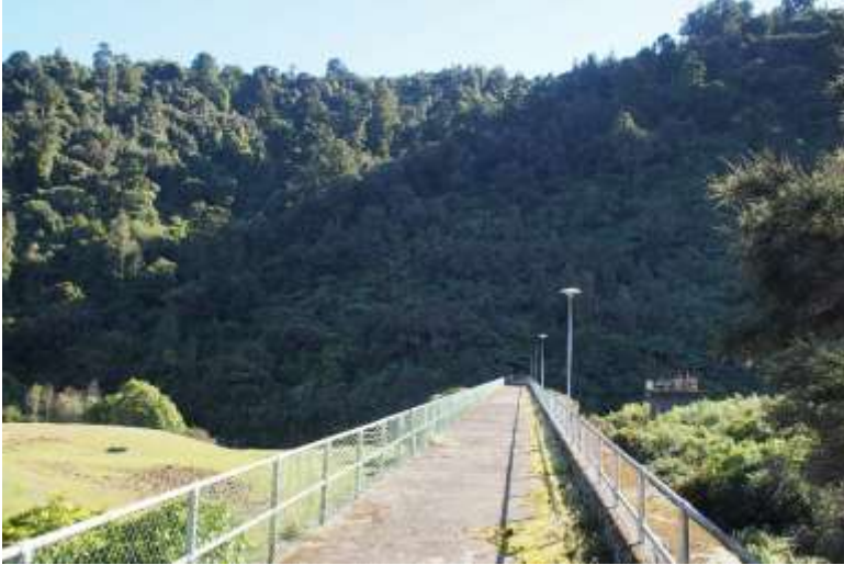
Photo 4: Western Spur from dam wall.
