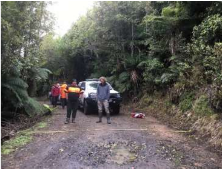
Photo 16: Existing access track at eastern ridgeline. Formed width is 5.9m. Lengths of this track will require widening to provide for both large vehicles and the fence.
