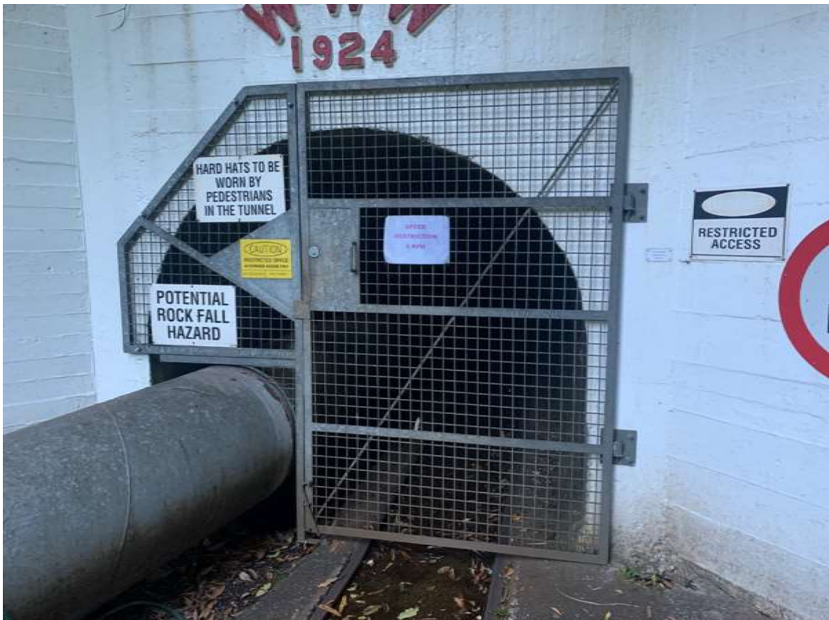
Figure 15. Orongorongo tunnel. Photo Ricky Clarkson
